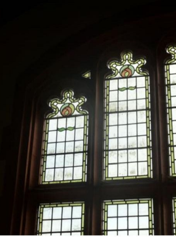
Interior view of south window
