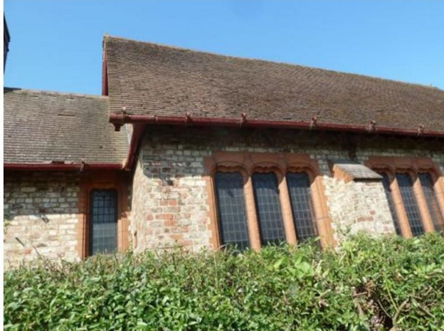
Eastern view of the building showing window detailing.
