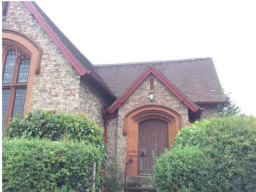
Front entrance doorway.
